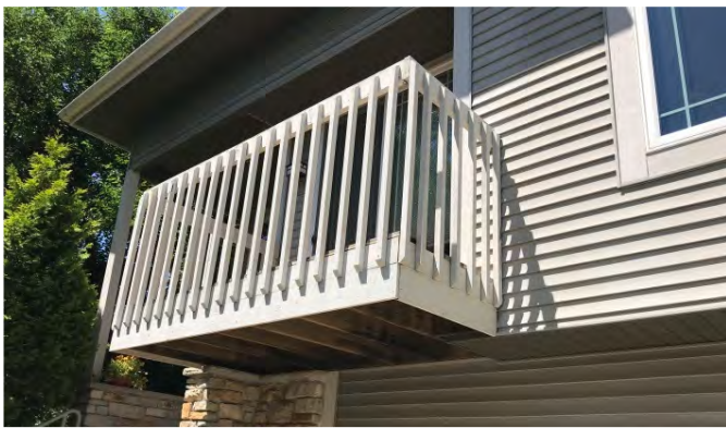
Townhouse Unit balcony with painted fascia, railing and balusters. (photo: Siebers)
