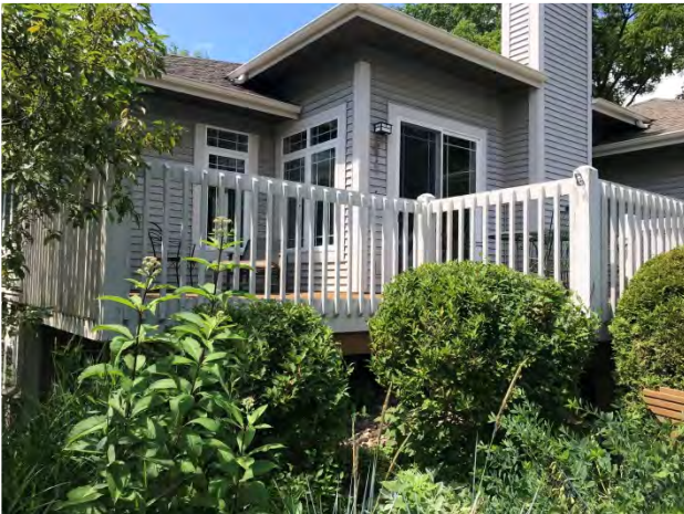
Small Ranch Unit side deck with painted railing (photo: Siebers)
